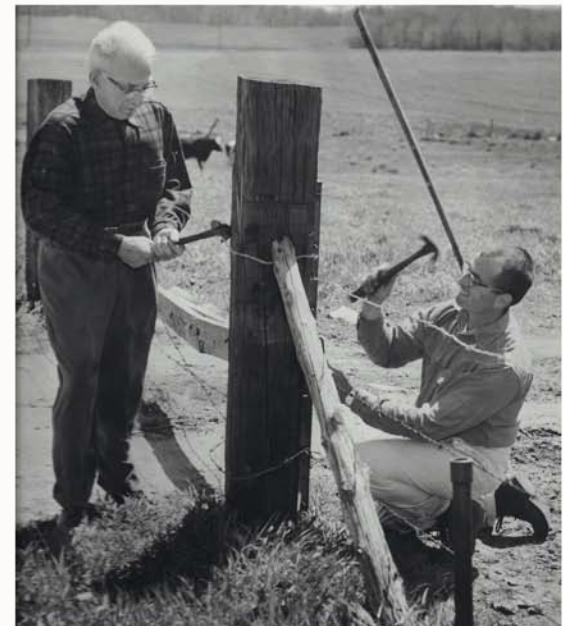
Floyd and Steve building a fence
